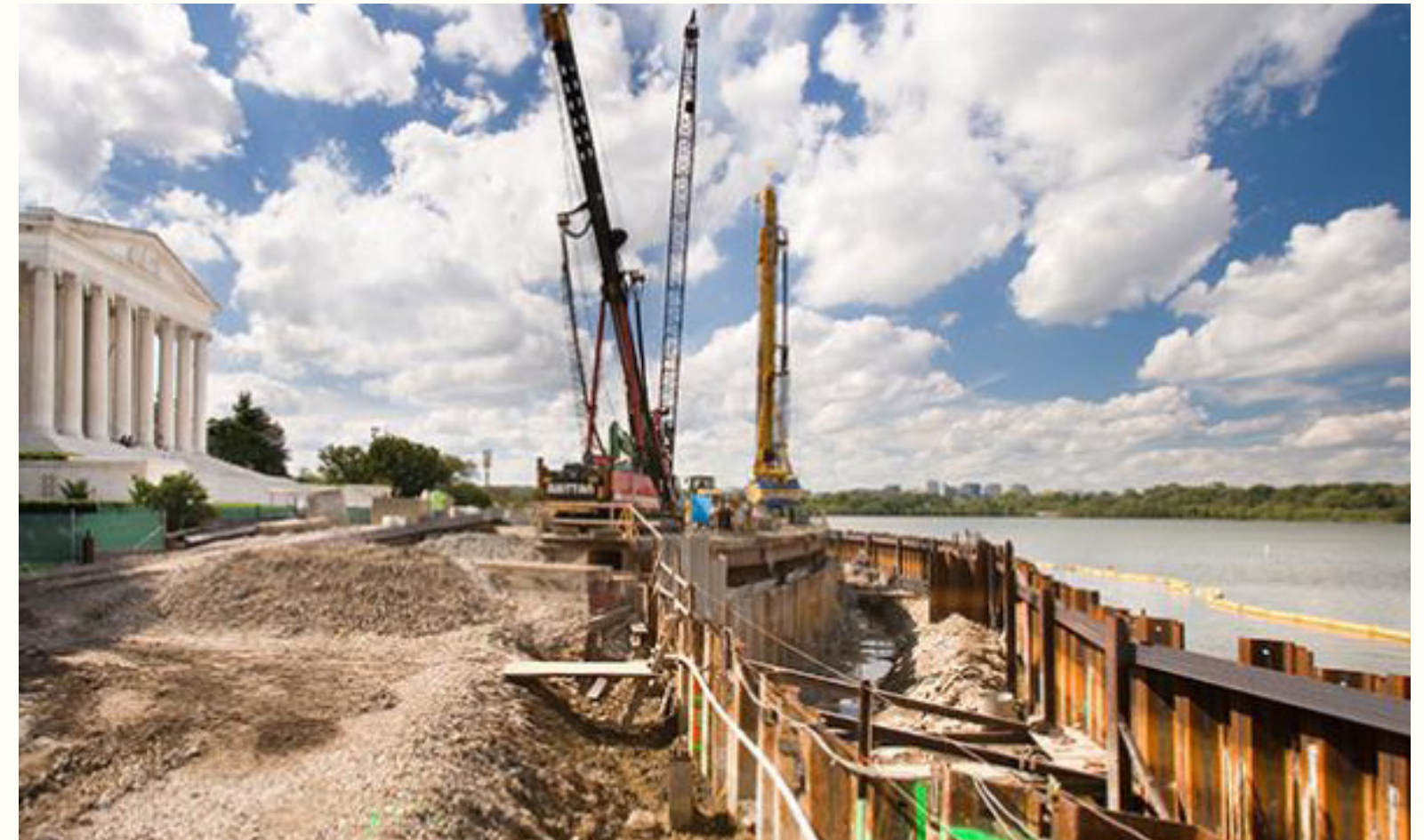
Figures 2.7 + 2.8 Seawall Restoration repairs to the Jefferson Memorial's sinking plaza at the northern shoulder of East Potomac Park (Trust for the National Mall)
