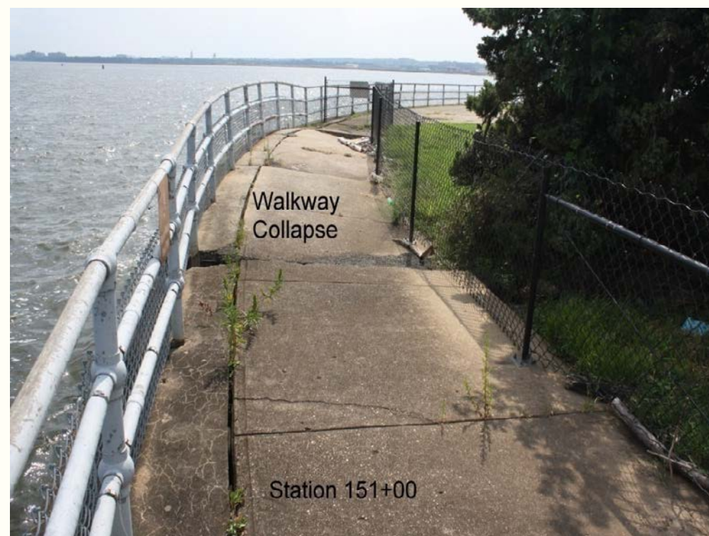
Station 151+00 Walkway Collapse, Washout under Slab
