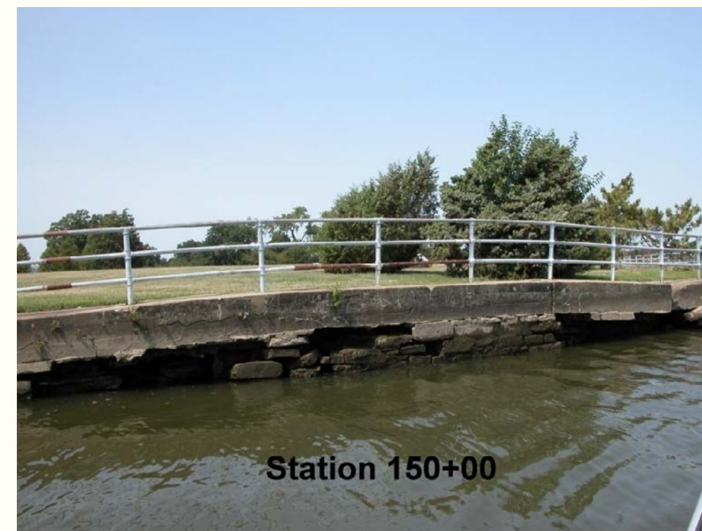
Station 150+00 Wall Collapse, Washout
